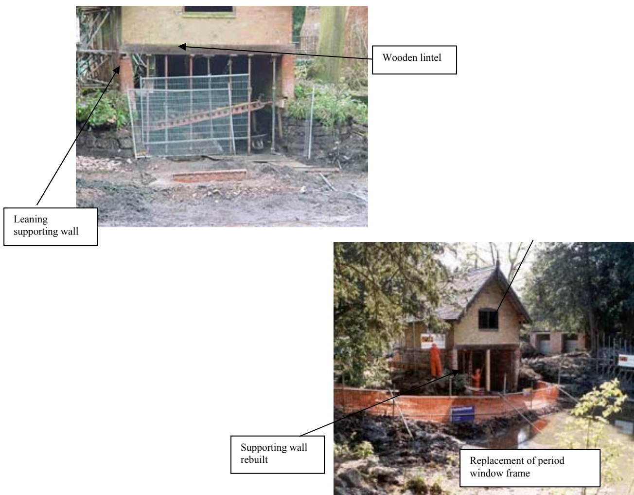
Figure 9.2.2 Restoration in progress
